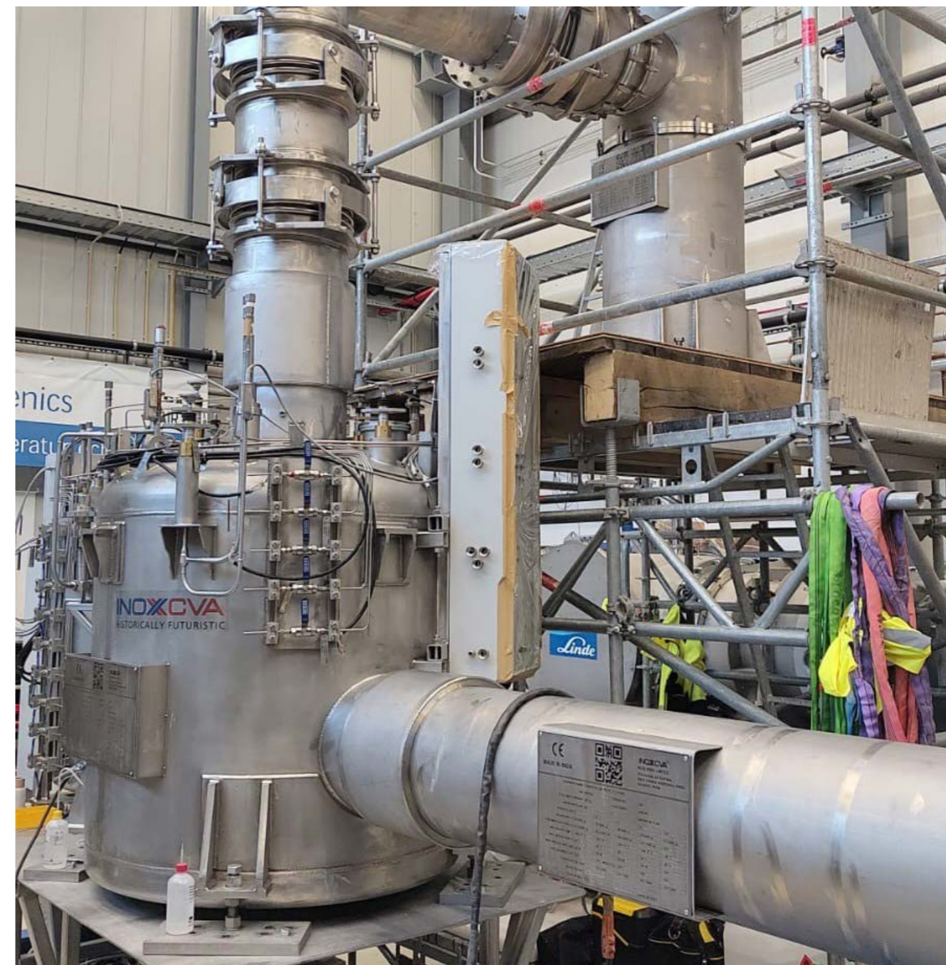
Installed image of Feedbox, Jumper and Transferline at FAIR Project
